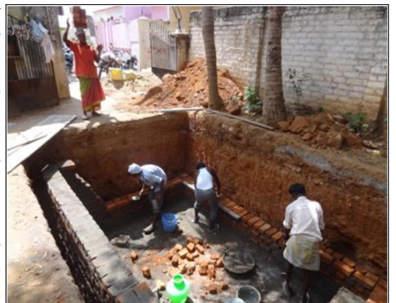
Construction of the water storage tank gets underway.
