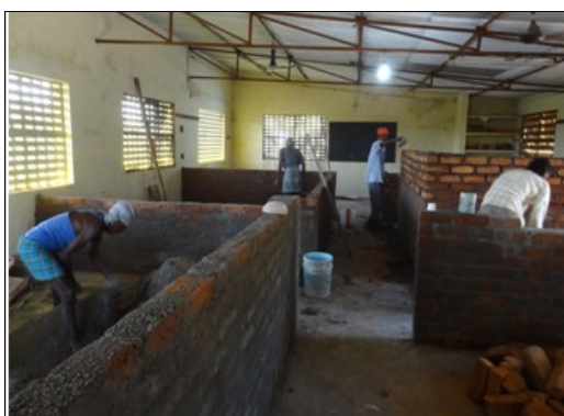
New bedrooms for the girls under construction.
