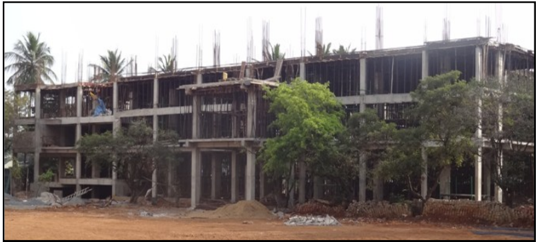
New classrooms and an auditorium/sports hall for Montfort School.
